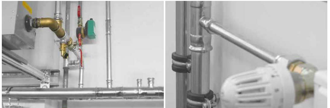
Examples of KAN-therm Steel installations
